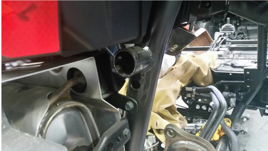
Figure 3: The two top mounts should weld to the frame as pictured.
